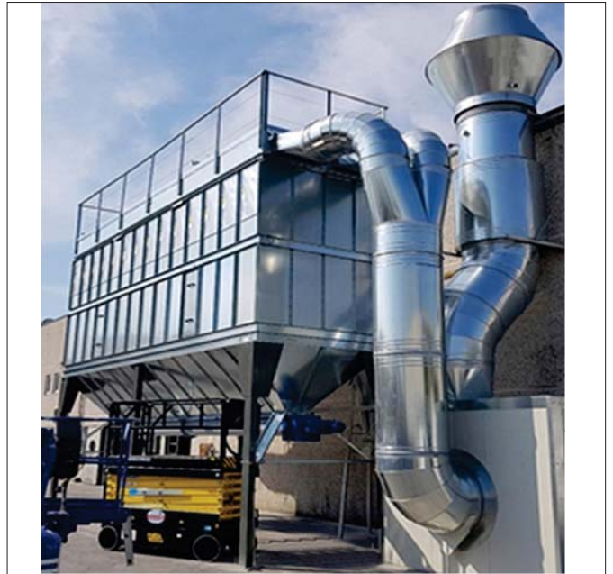
BERF 42 120 2500 1 T with screw and extraction fan in acoustic booth
